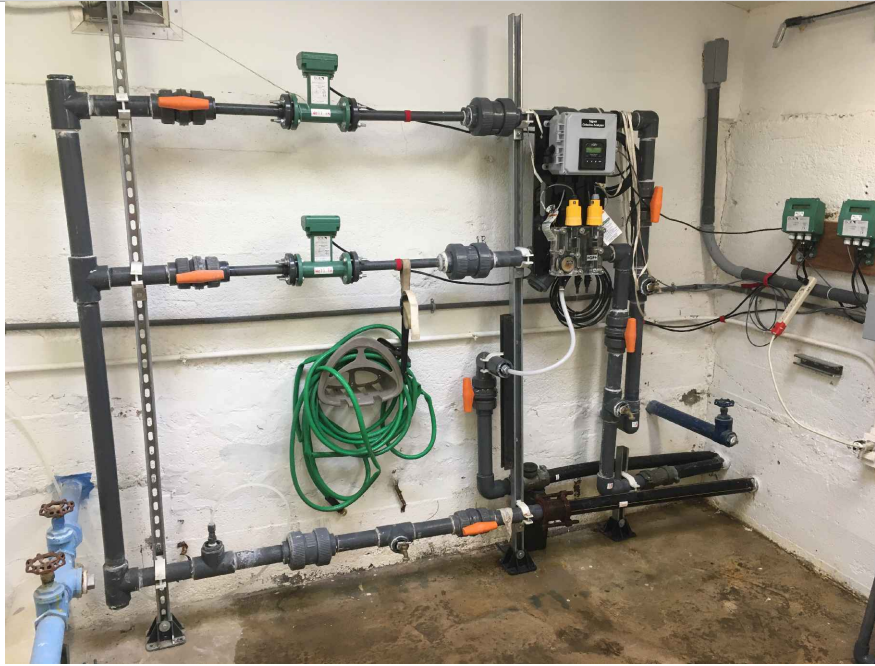
Photo 2 - Upper Treatment Building Interior Figure 1
