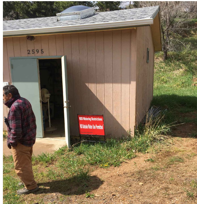
Photo 4 - Forks Treatment Building Exterior Figure 1
